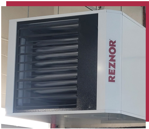
Ongoing HVAC repairs and replacements in 2022!
