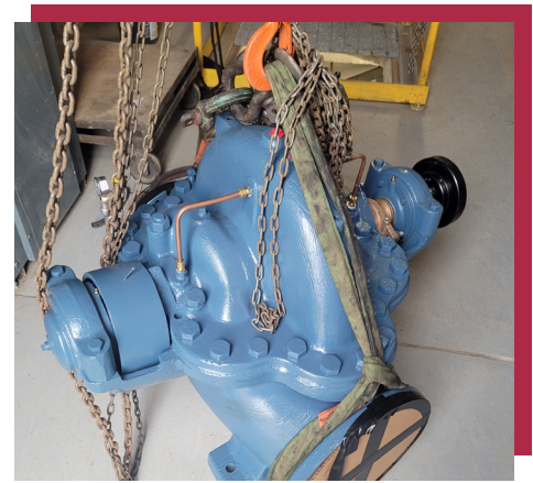
One of four High Service Pumps that maintain our water pressure and water supply located at the Filtration Plant.
