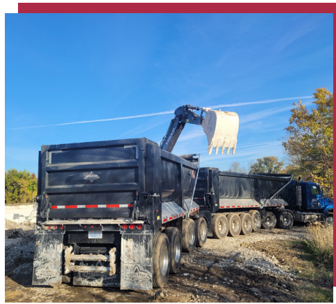
Each year used lime sludge is removed for beneficial use on farm fields.
