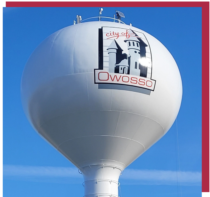
The newly painted West Tower!
