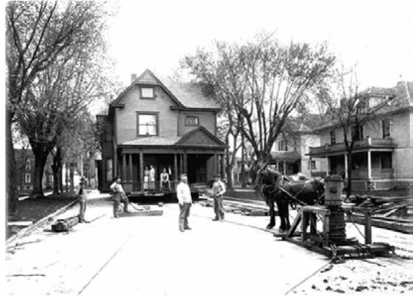
House Moving on Exchange Blvd. - house1.JPG
