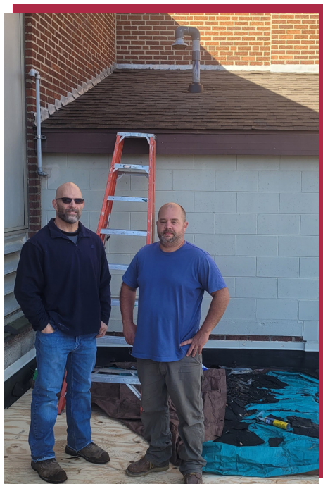
Saving funds by staff replacing a shingle roof.
