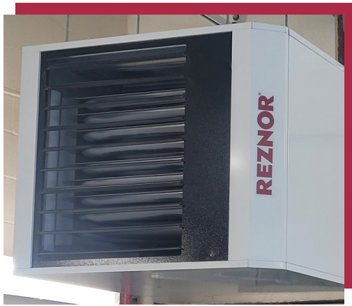
Ongoing HVAC repairs and replacements in 2022!
