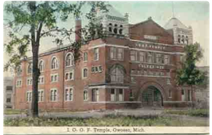
Old Armory on Mason Taken over by Oddfellows - Owoioof.JPG
