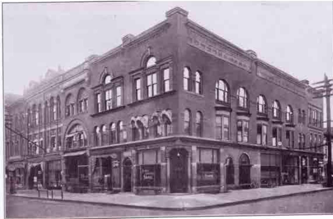
Citizens' Savings Bank Building, Southwest Corner of Washington Avenue and Exchange Street.
