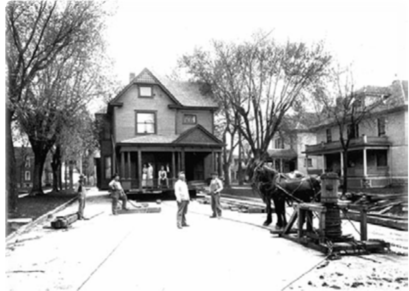
House Moving on Exchange Blvd. - house1.JPG
