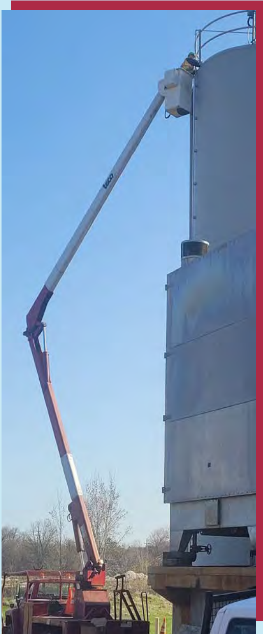
Service and replacing equipment using the DPW tree truck!
