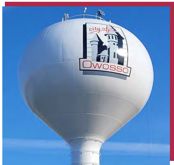
The newly painted West Tower!
