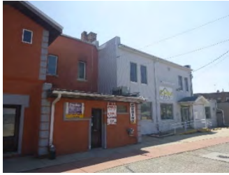
Building before, above (light colored building)
