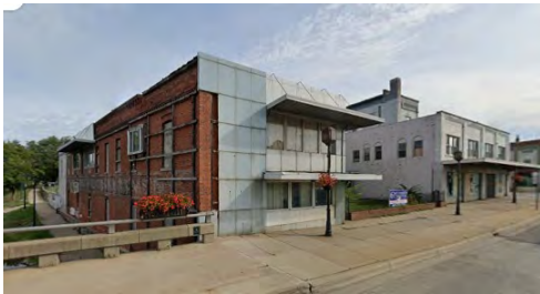
View from southwest 2019
