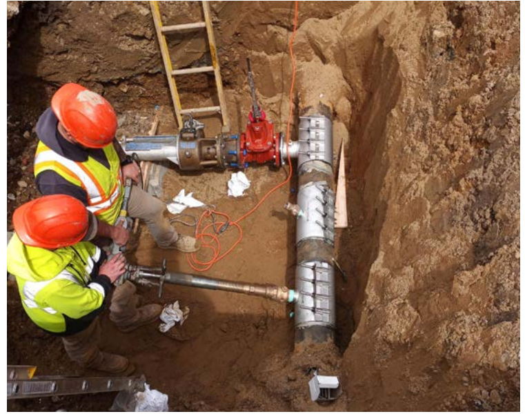
Large service being installed downtown
