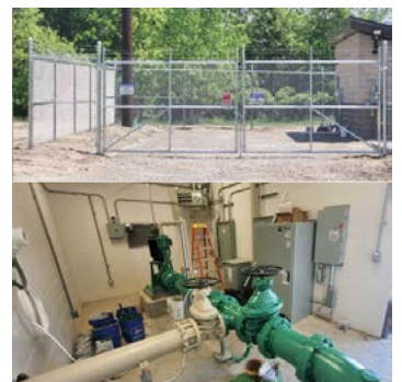
Inside and outside of new well building to be completed in 2024
