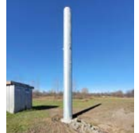
Communication tower base being installed at the WTP
